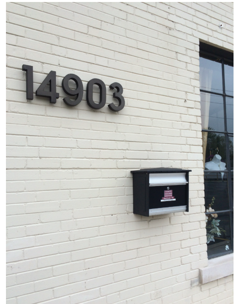
South Elevation of Building where mailbox is located.
